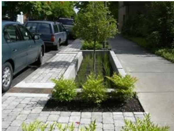
Figura 21 - Calçada na SW 12th Avenue Green Street, Portland, Óregon
