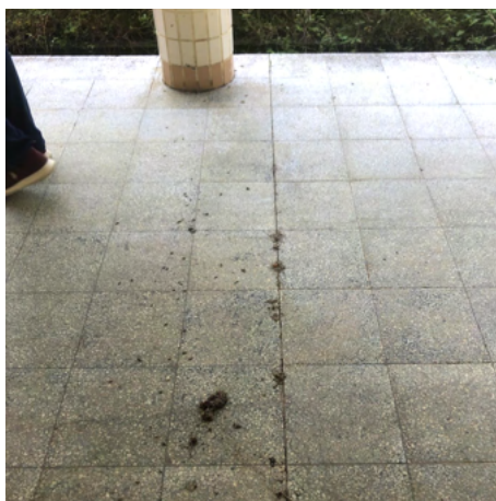
Figura B.16 – Fissura T8 (14/07/2021)
