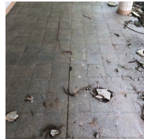
Figura B.46 – Fissura T24 (14/07/2021)
