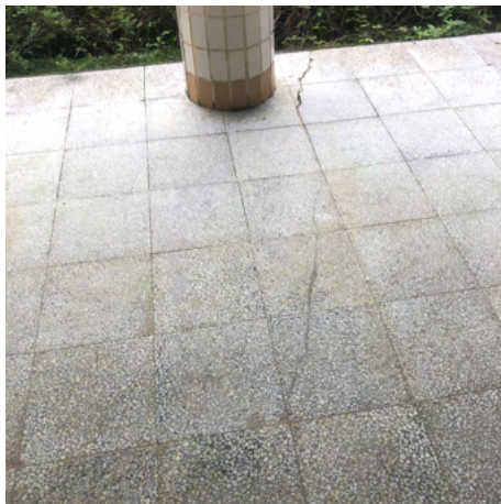
Figura B.20 – Fissura T10 (14/07/2021)
