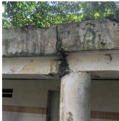
Figura B.44 – Fissura T23 (14/07/2021)
