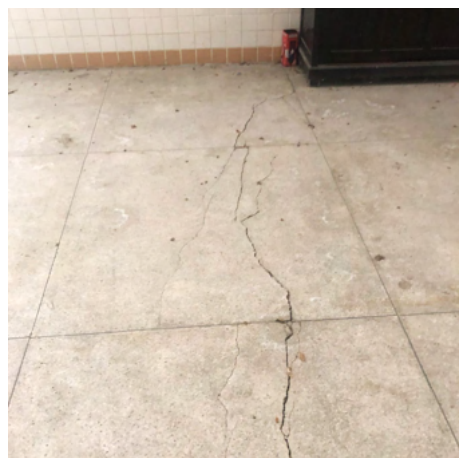
Figura B.14 – Fissura T7 (14/07/2021)
