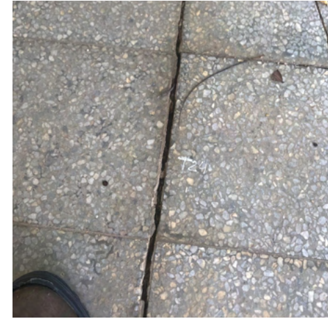
Figura B.46 – Fissura T24 (14/07/2021)
