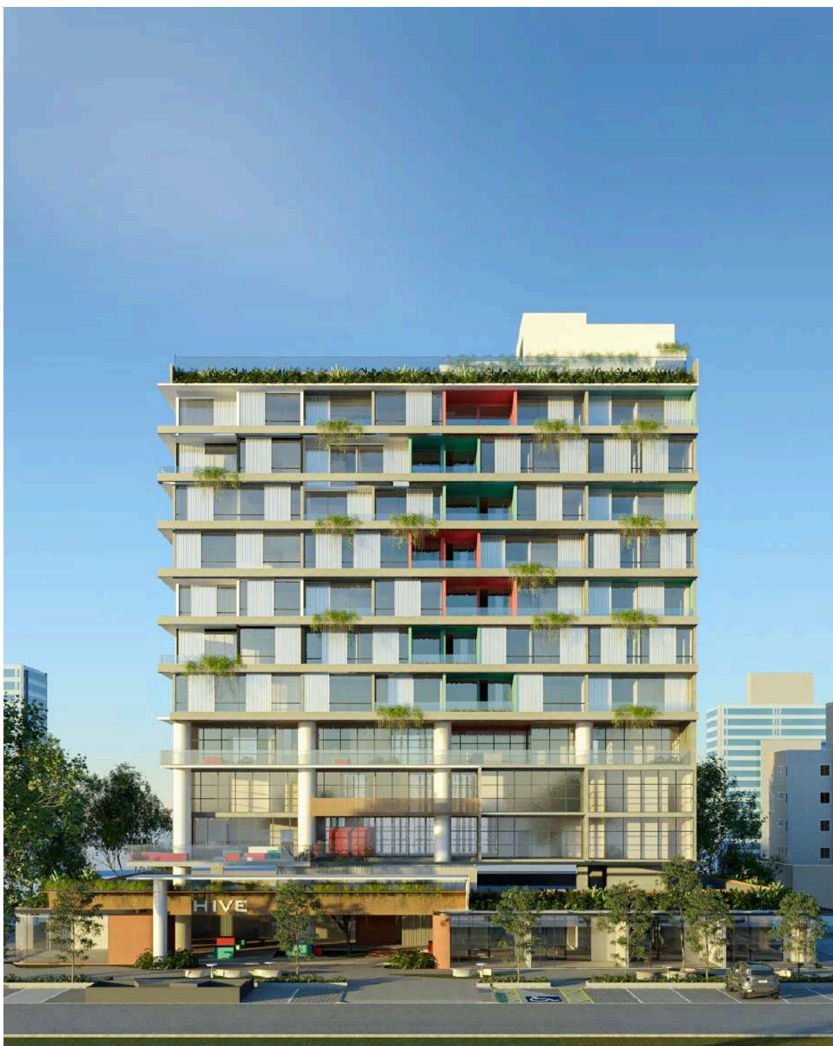
Figura 72: Fachada principal HIVE
