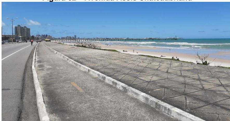
Figura 62 – Avenida Assis Chateaubriand
