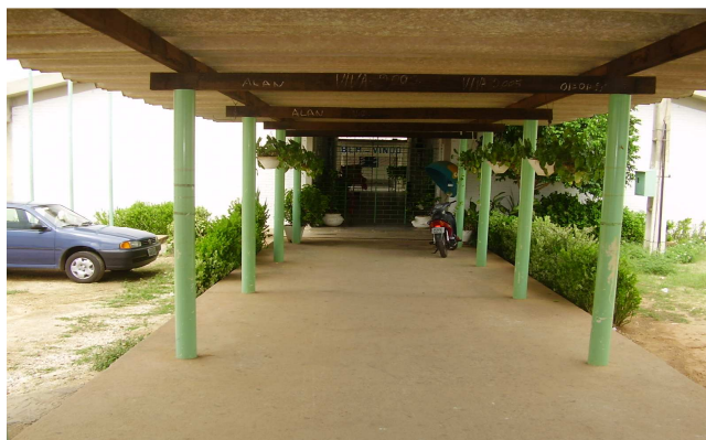
Picture 2: Main access to the school halls
