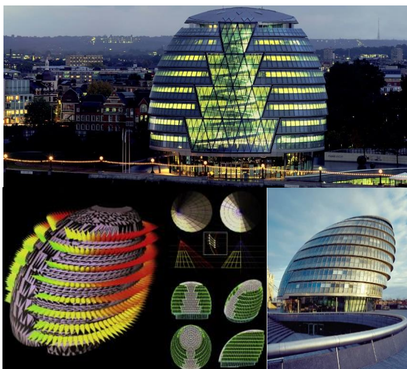
Figura 11 - Greater London Authority Headquarters building(FOSTER, 2002)
