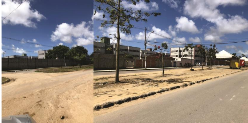
Figura 50: Muros perimetrais do conjunto Village das Artes.
