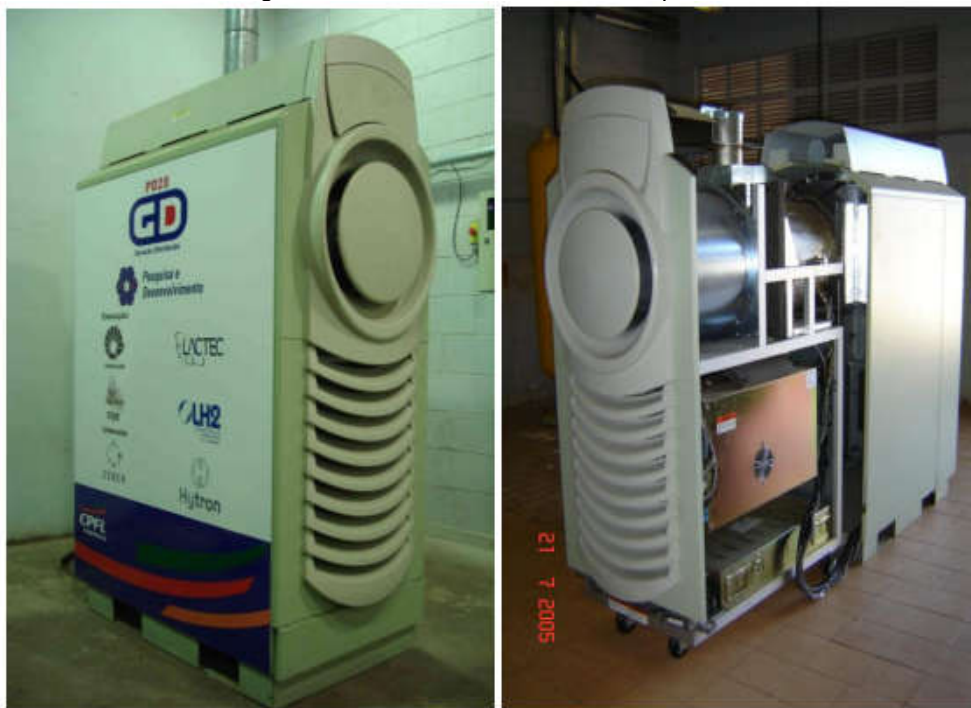
Figura 2.8 - Microturbina de 30KW Capstone.
