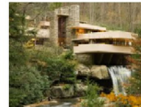
Flood Causes Damage of Frank Lloy... architecturaldigest.com
